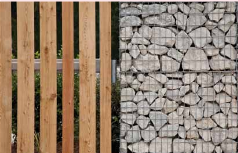
At the entrance of Val Semnoz shopping center, stones tightly encircled with wire mesh, remind clients the surrounding mountainous environment.
