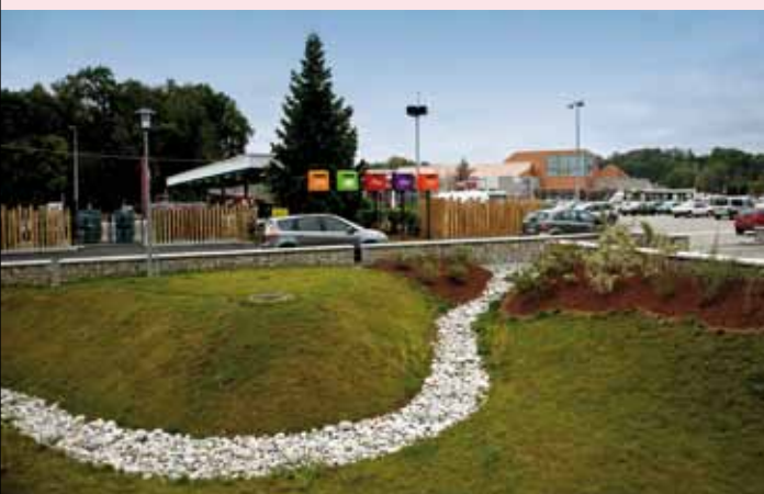
The rain garden is a natural filter that limits flood risks on the parking and partly cleans up wastewater.
